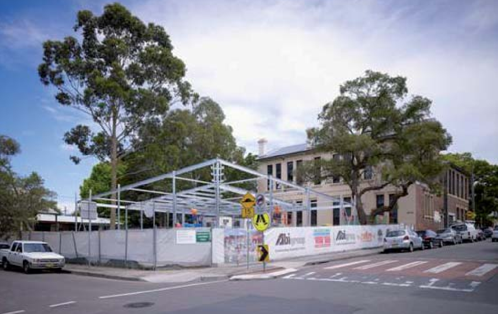
Infants School Newtown Construction Site December 2010
